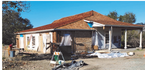
New roof is fire safe & historically accurate
