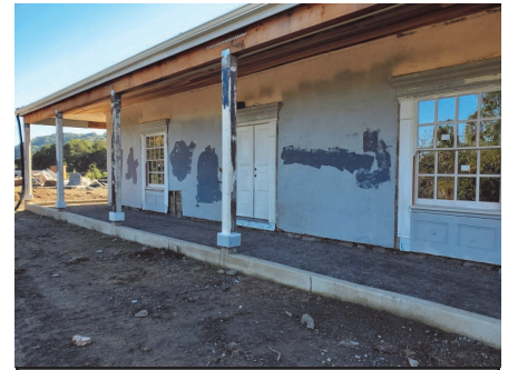
Front porch, new windows, reconstructed trim - November 2022
