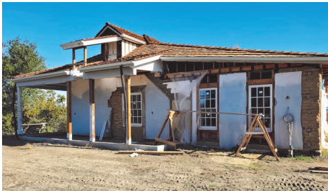
Reconfigured Attic Access
