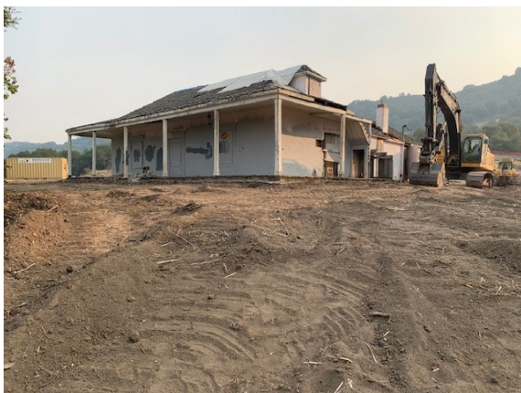
October 2020 Adobe Restoration
